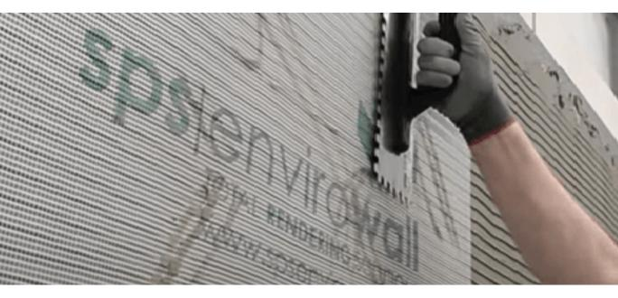
Our reinforcement mesh is the unsung hero of the render-only or EWI system. The mesh provides reinforcement and stability to the render, thus creating a perfect base for the subsequent application of an **SPS Envirowall** finish product.
