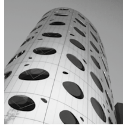
Futuristic architecture with an outer skin made of ALUCOBOND®: the Hotel Lindner Seepark in Klagenfurt, Austria
