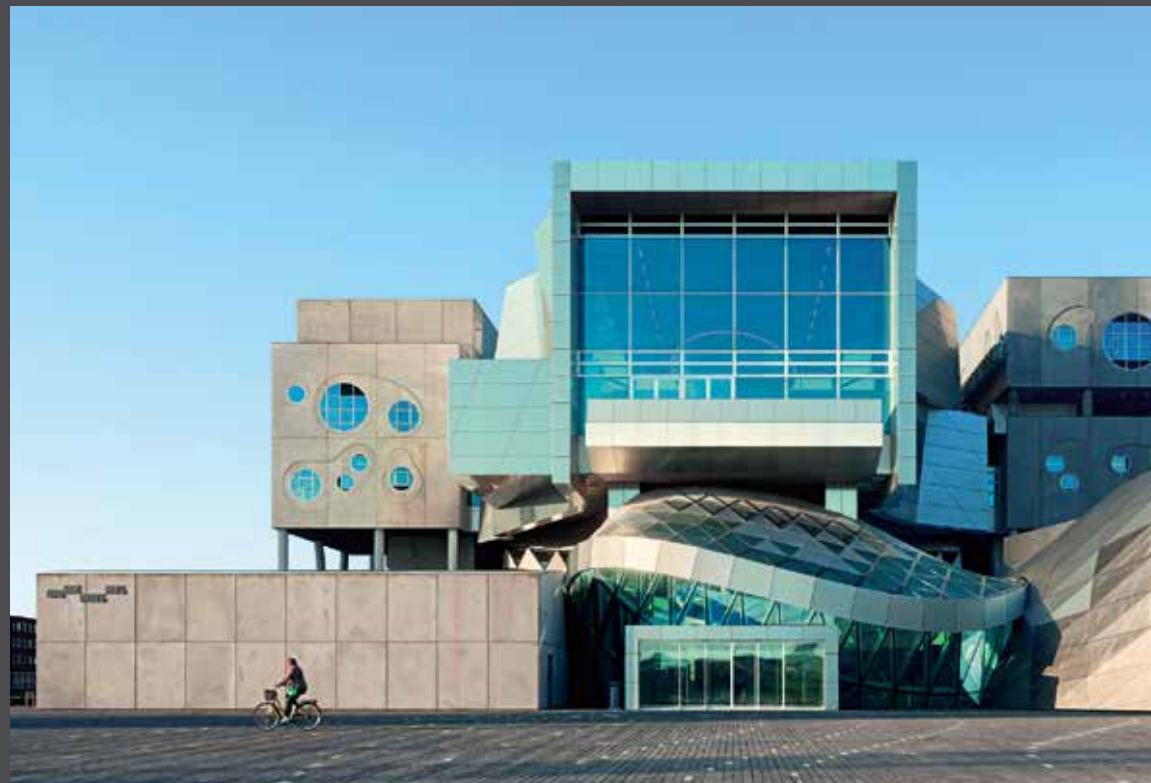
The ALUCOBOND® composite panel façade in naturAL Brushed gives the building its distinctive character. | Pictures: Duccio Malagamba
