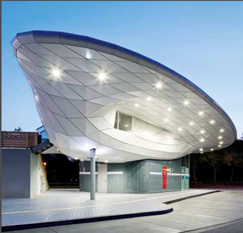
Poppenbüttel Bus Station's floating wing-shaped roof, made of ALUCOBOND® pure white. | Picture: archimages
