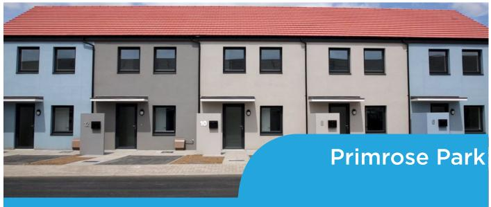
Client: Plymouth City Council • System: Wall System 2 • Material: EPS, Silicone Render Sector: Residential, Low Rise • Build Type: Masonry
