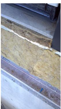
The use of screen or mesh is not compulsory. In a properly designed cavity there is for most time an air draft prevailing, which is not attractive for the presence of insects.
