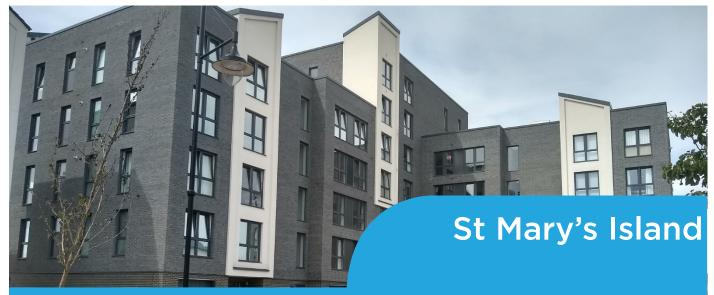
Client: Countryside • System: TS Rail • Material: EPS, SpeedySlip Brick Slips, Sllicone Render Sector: Residential, High Rise • Build Type: New Build
