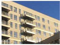
The appearance of the build was required to be of a classical upmarket style utilising concrete panelised cladding with trims and a sandstone colour render.
