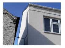
The addition of a new porch had to ensure no cold bridging occurred, this was achieved using an internal board to overlap.
